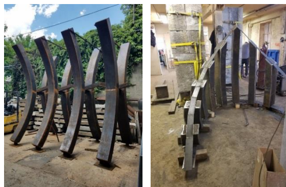
Sculpture restoration in progress
